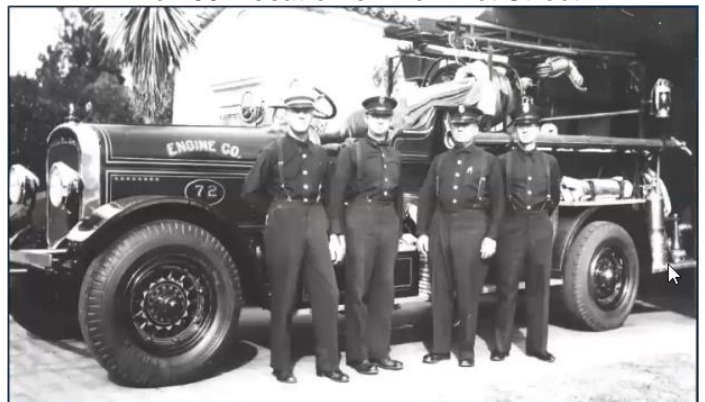
Canoga Park Fire Station: 1931 to 1978 (SEAGRAVE 750 GPM Pumper)
